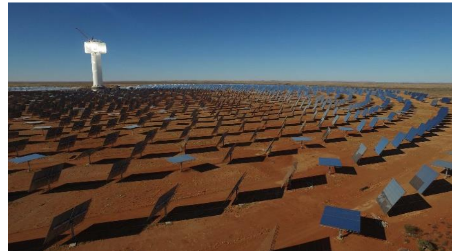
50 MW Khi Solar One heliostat field (Abengoa Solar 2016)
